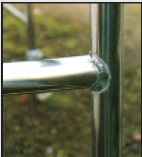
Saddle cut rungs for strength to eliminate frame racking problems.
