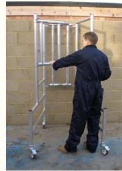
2) PULL GATE OUT BEFORE FITTING PLATFORM
