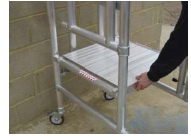
2 ) RELEASE PLATFORM LOCK BOLT AND LOWER PLATFORM OR LOCATE INDIVIDUAL PLATFORM
