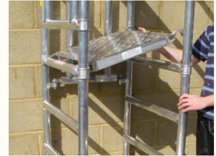
2 ) FIT PLATFORM AT REQUIRED HEIGHT ( 1200 SHOWN )
