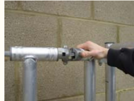
1 ) OPEN FOLDING FRAME AND MECHANISMS WILL LOCK AUTOMATICALLY
